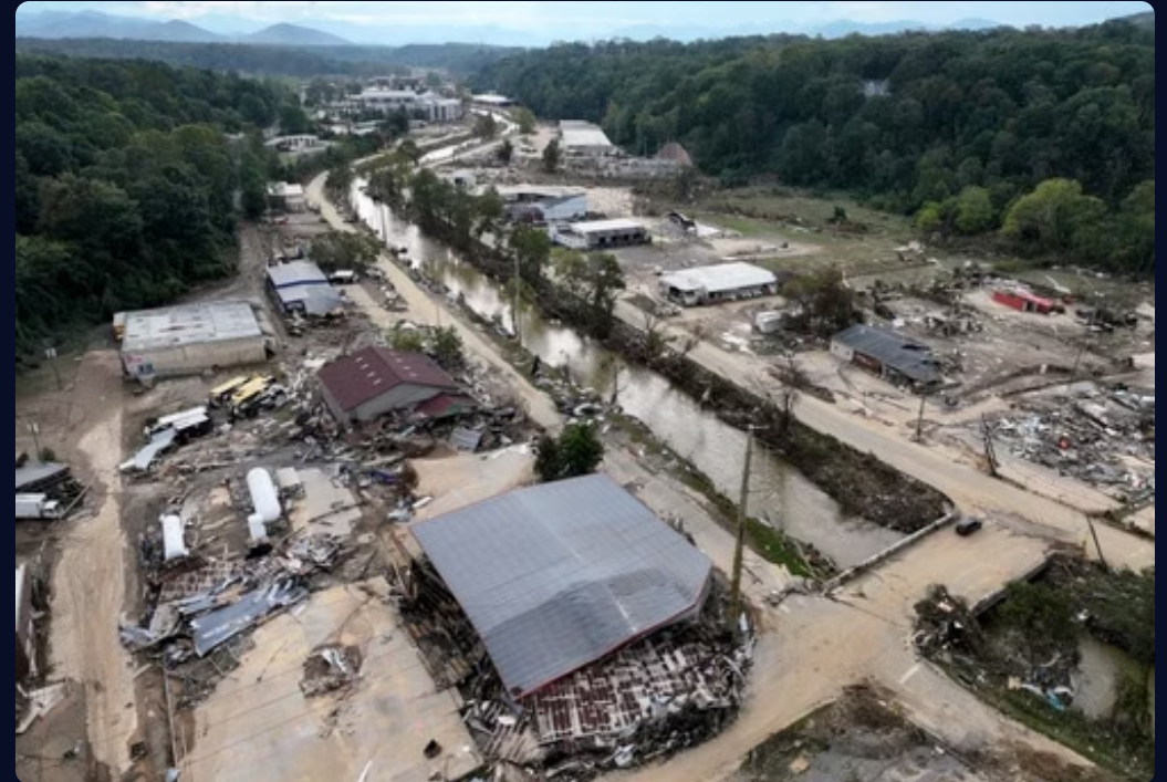
Asheville, North Carolina post Hurricane Helene
